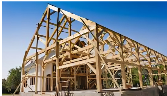
Fig. 3.1.7: structural framing timber
